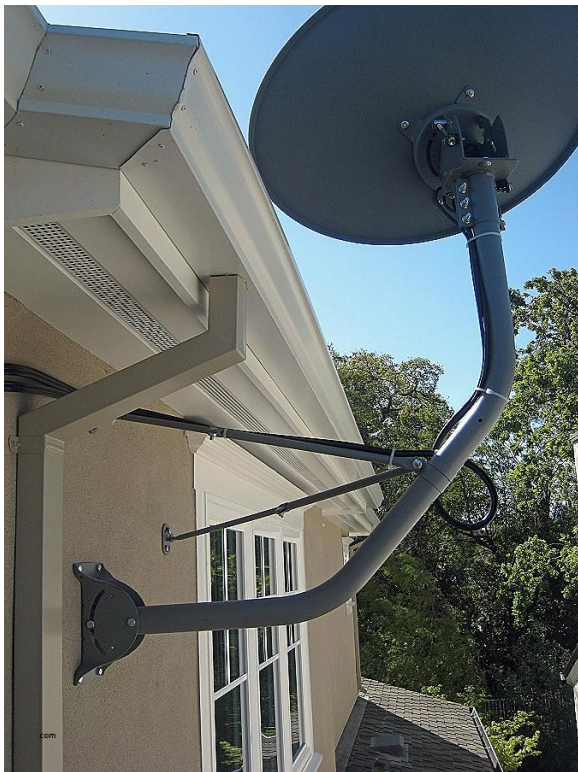
FIGURE 1. Acceptable wall mounted dish antenna
