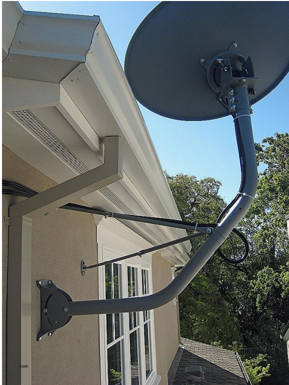
FIGURE 1. Acceptable wall mounted dish antenna
