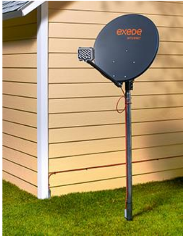
FIGURE 2. Acceptable pole mounted dish antenna
